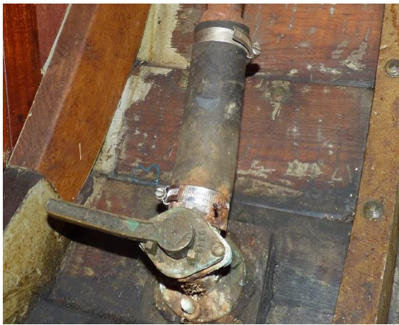
Corroded J-clip on sink waste
